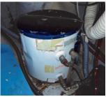
time, the boat will likely need a first or second replacement. Here is how a new marine Raritan 12 gallon heater is installed, considering the cramped quarters in the engine compartment and lazarette.
