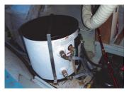
The new Raritan heater comes in by the reverse path. It has a plastic flange around the bottom instead of the four "L" brackets that mounted the old unit to the shelf. Regardless of the make, put in extra screws with fender washers. Strap the unit down with two pieces of plumber's tape\* over the top of the heater and down to the shelf. The photo was taken while trying to reuse the original strap setup. Best to make new straps. Galvanized plumber's tape\* was used which is available at
