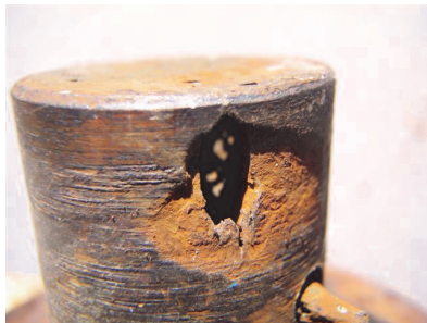
Light spots inside hole is sun shining through pin holes in top of pivot pin
