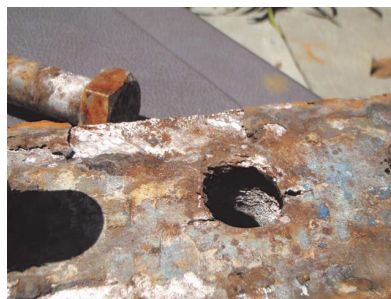
Corroded bolt hole
