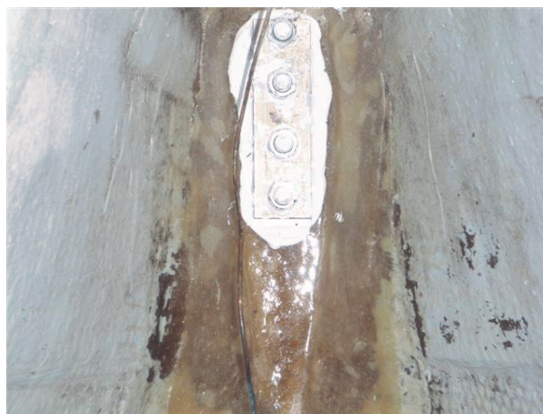
Finished installation from inside hull
